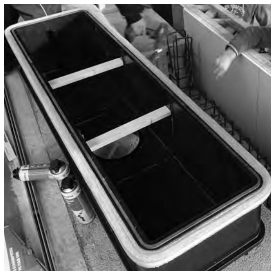
Image 3 BaduJet Turbo Pro - Foam Strip & Wooden Supports
